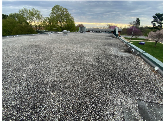
32 – BUILT-UP ROOF MEMBRANE
