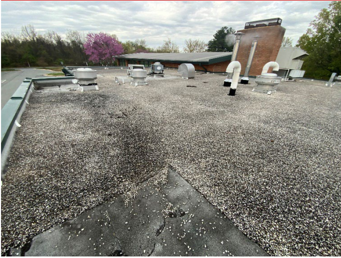
31 – BUILT-UP ROOF MEMBRANE
