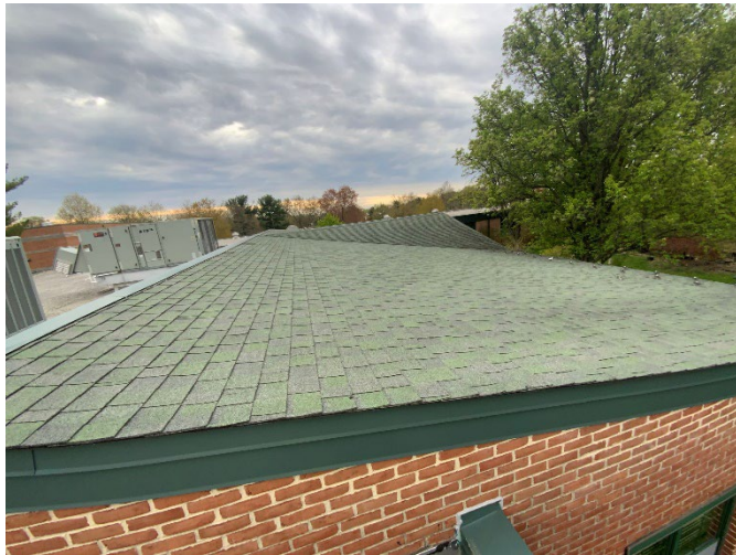
33 – ASPHALT SHINGLE ROOF
