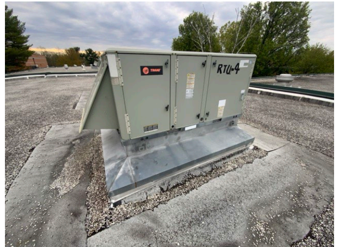
28 – PACKAGED UNIT AT ROOF LEVEL
